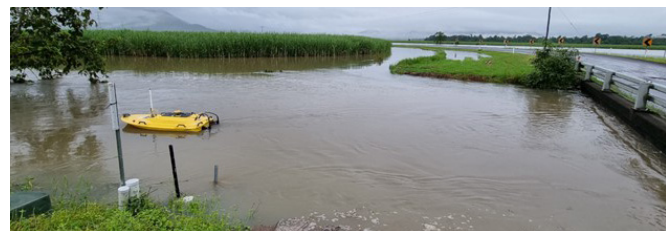
Figure 5. Bridge Deck at Tributary
