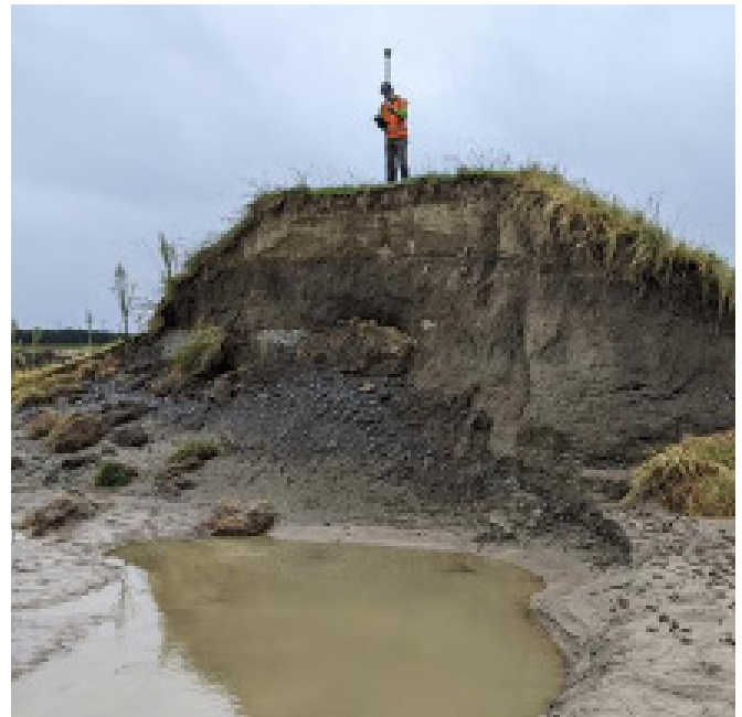
Change detection of flood extent using Sentinel 2 imagery (left); and manual survey of breached stop bank (right).
