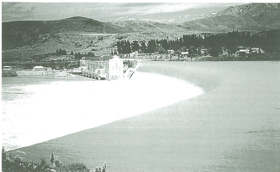
Figure 3.1. Waitaki Dam spillweir and powerhouse discharging “clean” flood water on 14 December 1995 (A Pattle).
