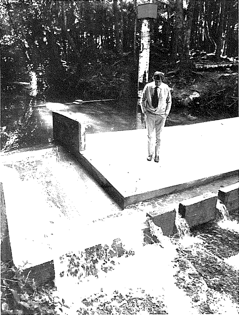
FIG.—3 Crump weir near Whangarei, New Zealand, with flow in the low-flow section only.
