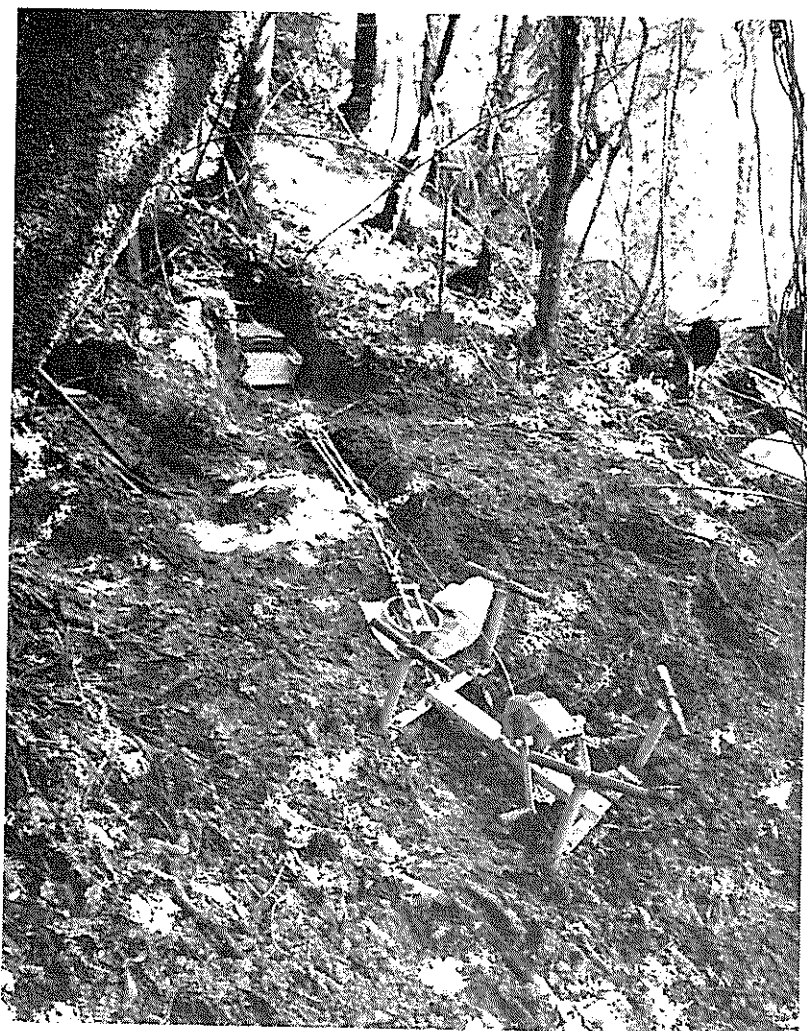
FIG.—1 An open side field shear box in use in a forested area with coarse soils. The force is applied by the winch and measured on the proving ring. The box is placed on an in situ excavated monolith and the normal load is applied by the weights on top of the box.
