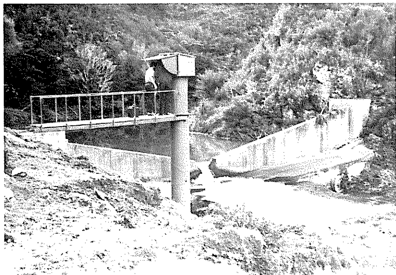
FIG. — 1 Compound weir, Northland, New Zealand.
