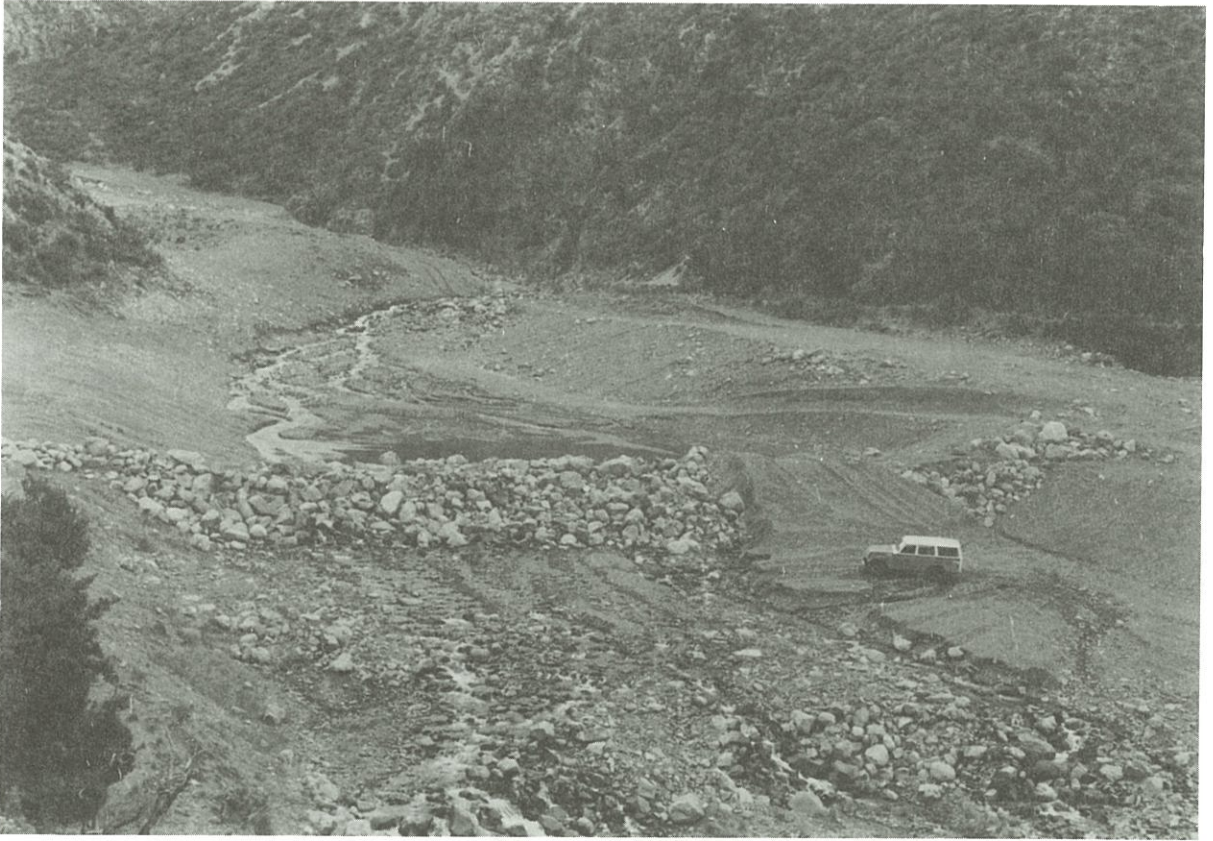
Figure 13.6 Sediment trap formed by permeable rock dam on Dry Acheron Stream, Canterbury foothills (photo I.E. Whitehouse).
