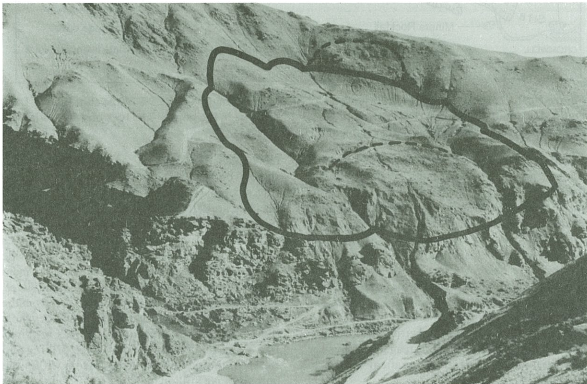
Figure 20.17 Aerial photograph of the Cairnmuir landslide in Cromwell Gorge. (Photograph: Courtesy of the Clyde Power Project, Electricity Corporation of New Zealand)
