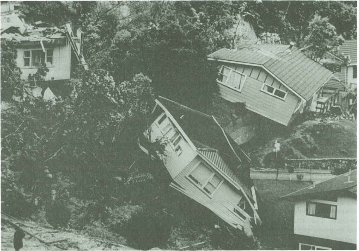
Figure 20.13 An intense rainstorm on the 20 December 1976 led to widespread landslipping in Wellington. While only one life was lost numerous houses suffered damage such as these in Stokes Valley. (Photograph: Courtesy of The Evening Post)
